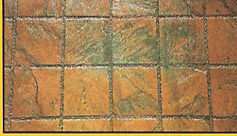
6" x 6" Slate Tile Grouted
