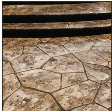
Flagstone imprinted concrete pattern was created using:
